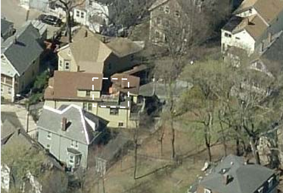
Existing deck that will be replaced indicated within white dashed box
