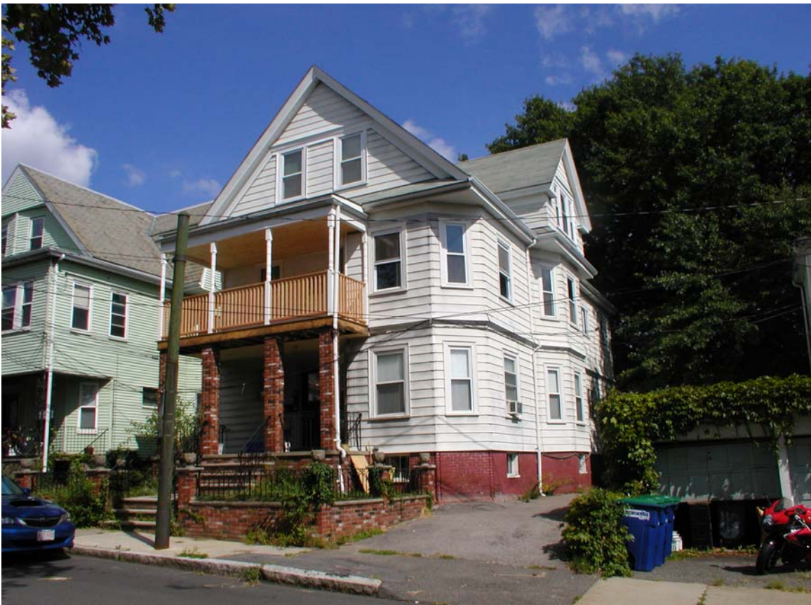
Existing Conditions: Front and Right Side Façades
