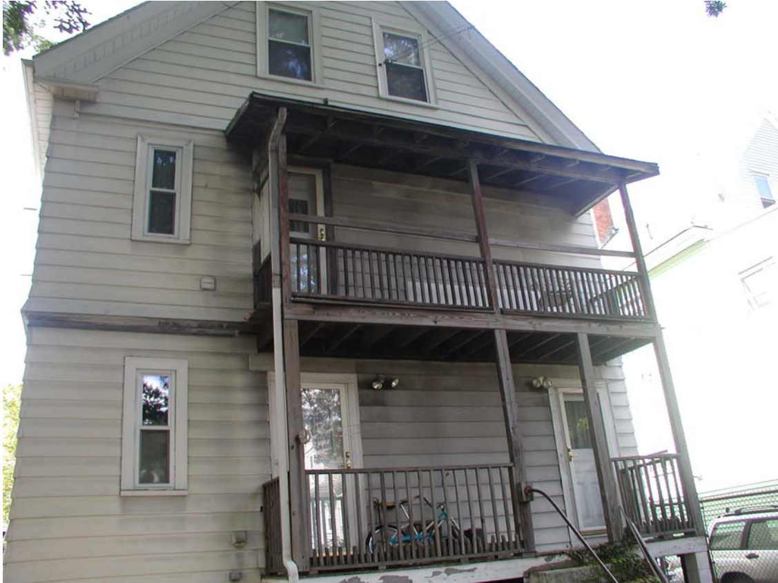
Existing Conditions: Rear Façade
